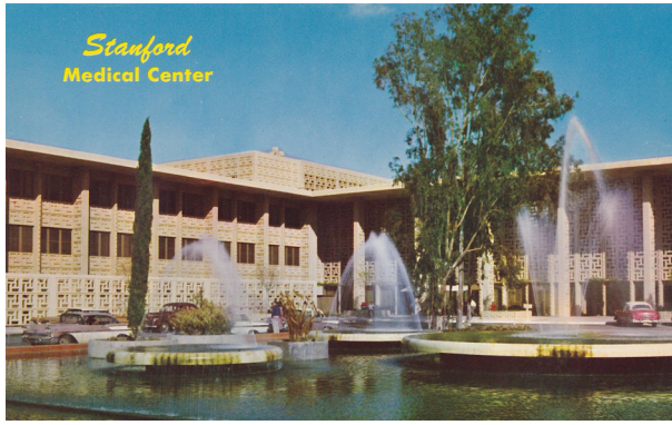
Figure 4. Stanford Hospital Palo Alto, opened in 1959.
